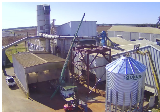
Construction of in-shell peanut holding bin
