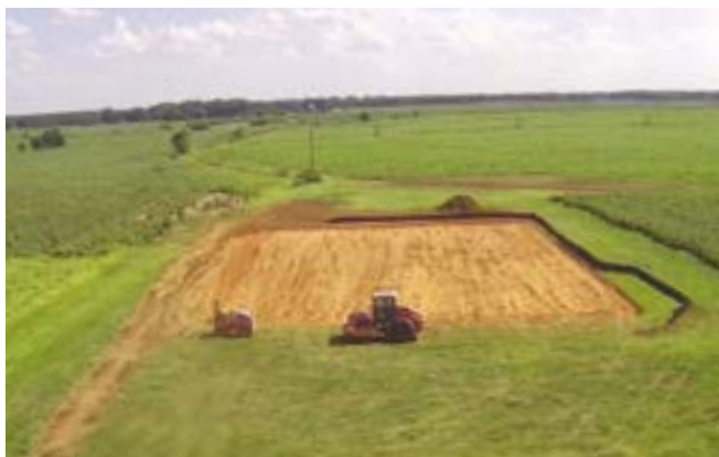
Beginning stages of construction for GSD cold room storage facility in Plains, GA
