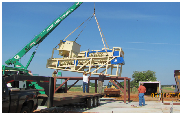
Lowering New Air-Gap Cleaner, Plains
